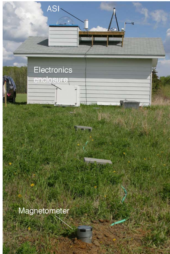
Fig. 13 GBO station as installed in Athabasca, Canada
